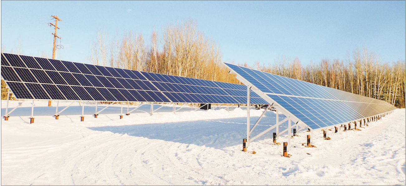
The expanded Fort Simpson solar array includes 178 new panels, bringing the total peak production up to 104 kilowatts.
