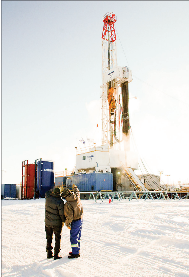
Sahtu elders get a tour of MGM Energy Corp.'s camp and drilling project near Tulita on Feb. 13.
