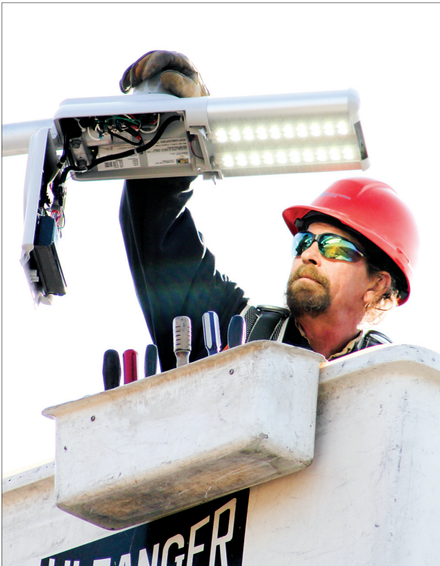
A Northland Utilities worker installs a set of new LED bulbs on one of Yellowknife’s many street lights.
