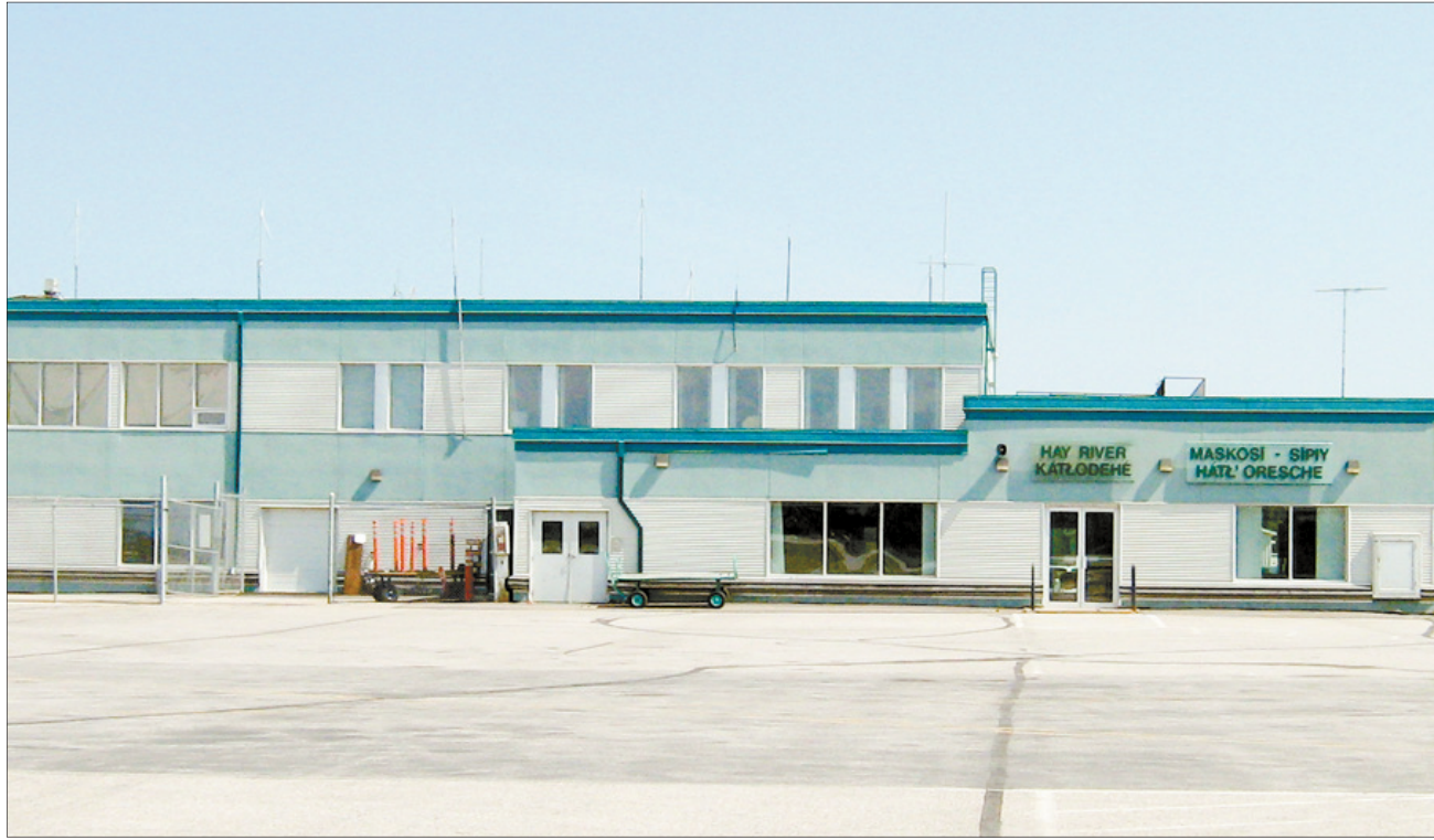
The runway at the Hay River airport is scheduled for new repairs sometime this summer.
