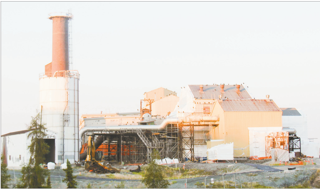
Mid-summer progress highlights the brick-by-brick take-down process.
