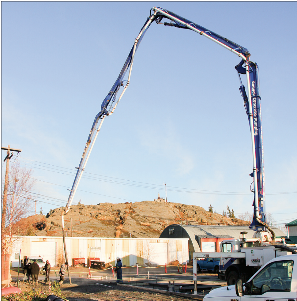
Work crews pump cement for a picnic area on Yellowknife's Government Dock.
