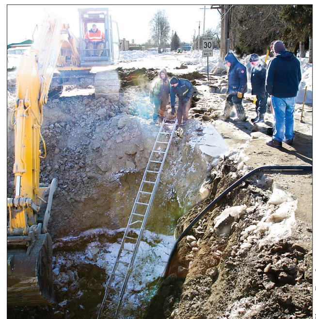
In addition to trying to repair old brittle pipes in cold weather and dealing with chunks of frozen ground, crews down in the excavation were dealing with mud as the flow of water mixed with the silt. That meant constantly pumping out the gritty mess and hauling it away by the truckload.
