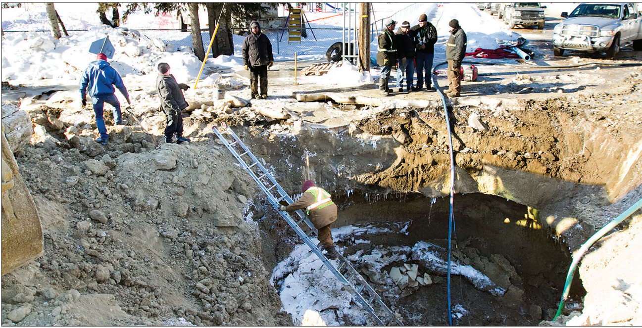
A mud filled crater adjacent to McDougal Rd. and close to JBT Elementary school has been the focus of attention for work crews with heavy equipment for over three weeks now as efforts in a troublesome water main break repair job are ongoing.
