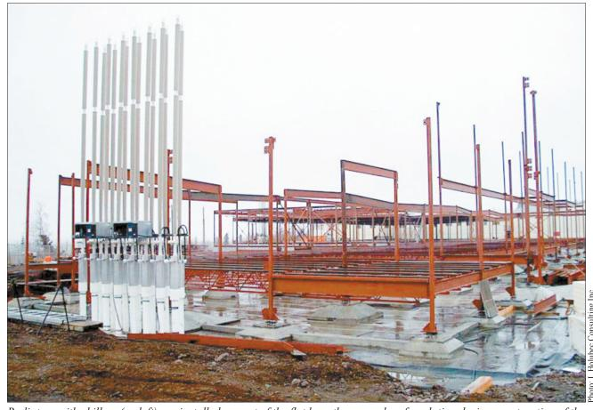
Radiators with chillers (on left) are installed as part of the flat loop thermosyphon foundation during construction of the Beaufort Delta Hospital in Inuvik. The hospital is one of several government buildings in Inuvik featuring thermosyphon technology, which aids in preventing permafrost degradation and the subsequent damage to infrastructure.
