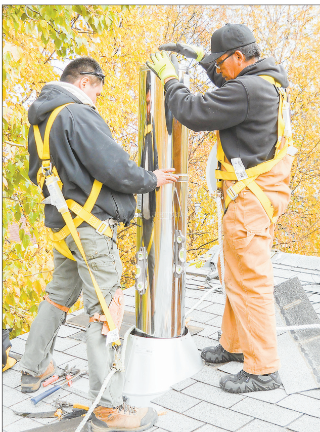
Donald Andre and Alfred Beaverho install a chimney on a home in Fort Simpson last fall. More and more NWT residents are choosing biomass fuel to heat their homes.
