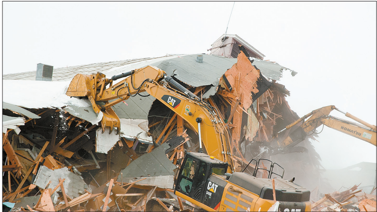
The demolition inspired mixed emotions from Inuvik residents.
