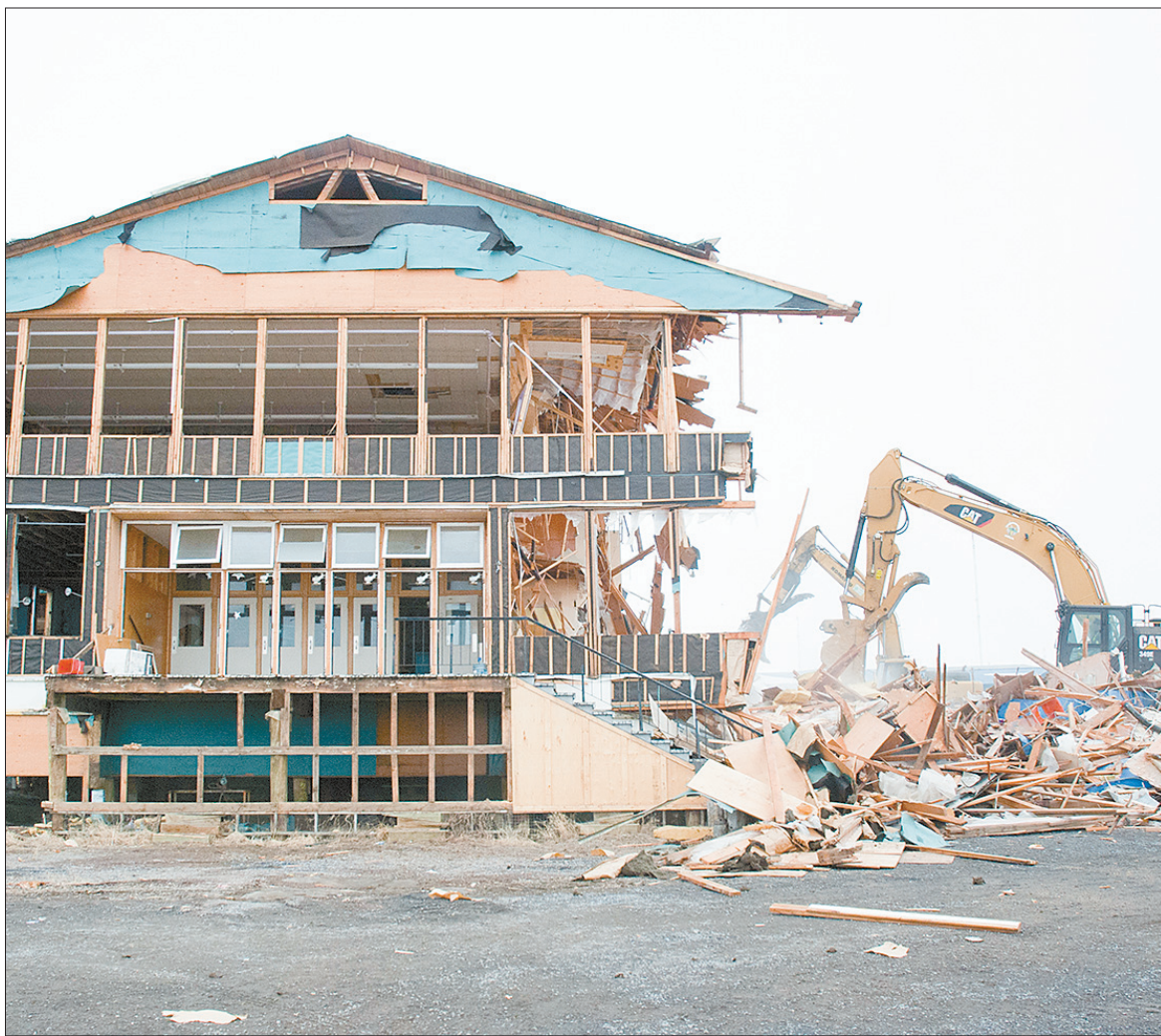
It took four excavators four hours to demolish Sir Alexander Mackenzie School in Inuvik last Friday.
