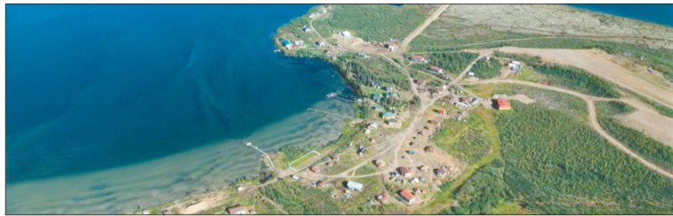
All residents and businesses in Colville Lake lost power last week after a line was knocked down.
